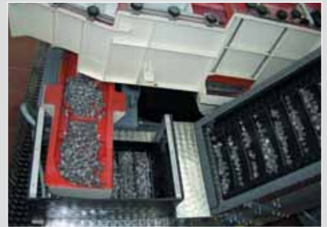
Lower cross-conveyor channel with residual water screen segment and media conveyor belt
