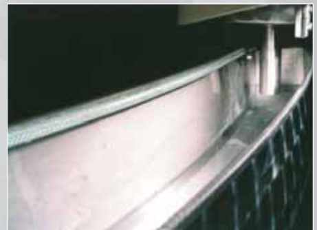
Dirty water discharge channel
